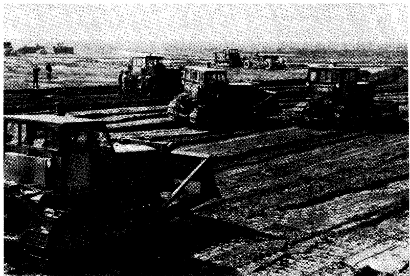
Shengli Oilfield airport under construction.
