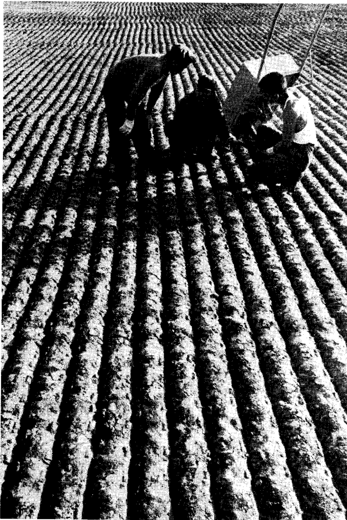
Testing the base surface for highway construction.
