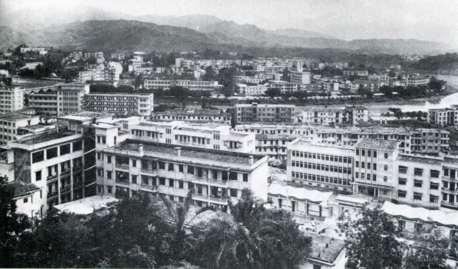
A glimpse of Tongza Town, Capital of the Hainan Li and Miao Nationality Autonomous Prefecture.
