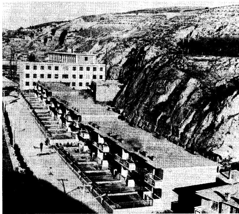
New two-storey buildings in Shangzhangjiafen village.
