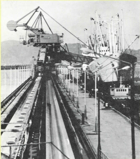
The 25,000-ton wharf in Beilun Port.
