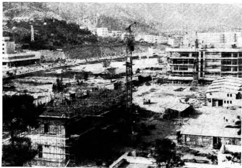
The Shekou Industrial District under construction.
