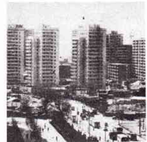
Beijing under construction. Photo by Zong Chao
