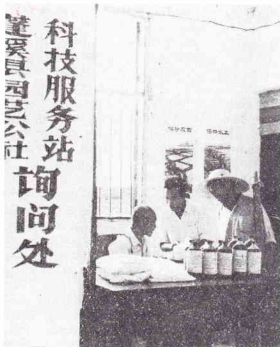
A commune scientific and technical service centre in Sichuan Province.
