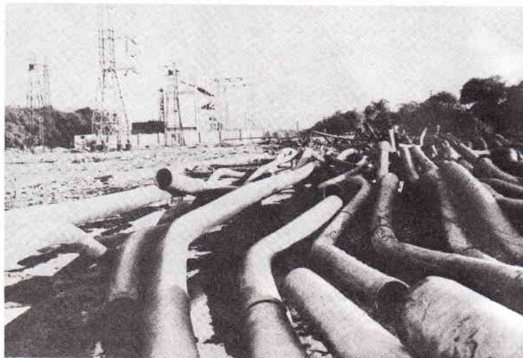
Iranian oil pipes were damaged.
