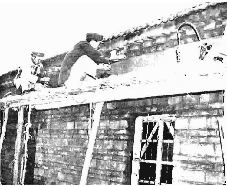
Peasants building new tile-roofed houses.
