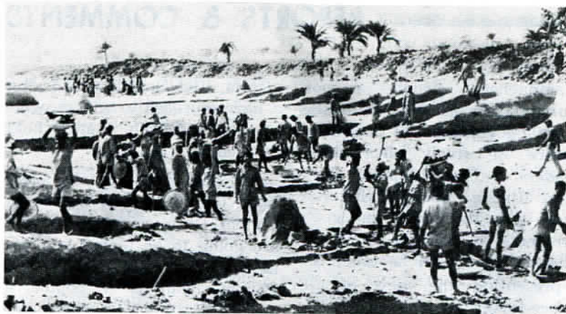
Building a canal in Bangladesh.
