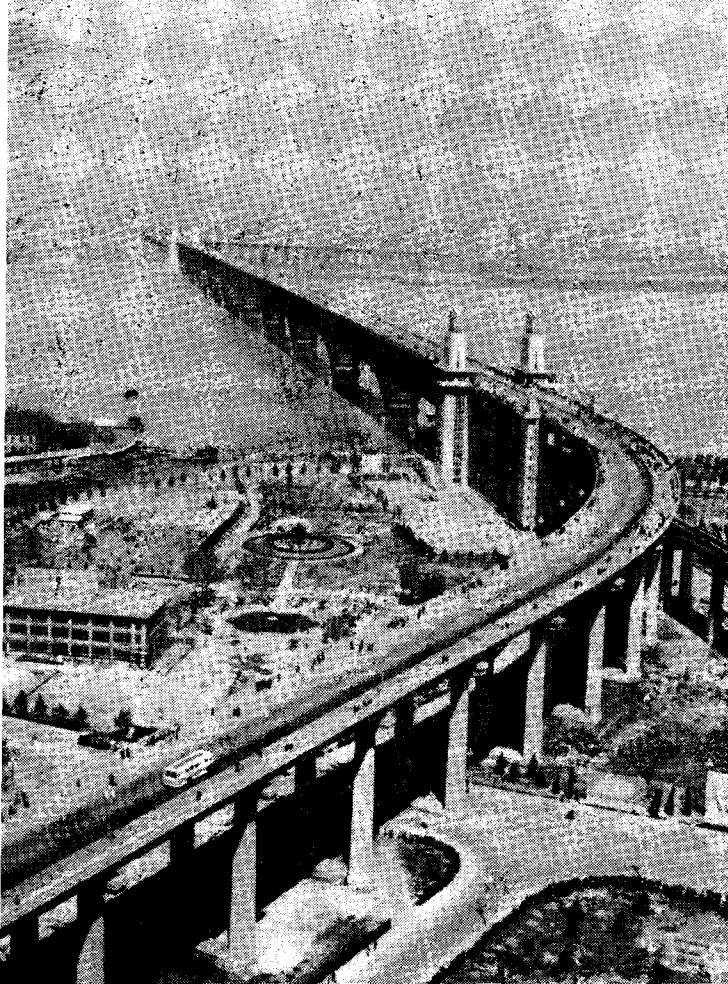
The Nanking Yangtze River Bridge.
