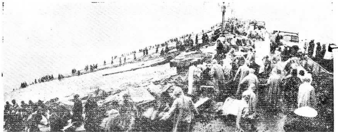
Reinforcing the Paiho River dam of the Miyun Reservoir on Peking's outskirts.
