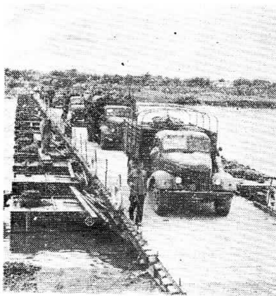
Commanders and fighters of the P.L.A. putting up a pontoon bridge to enable relief materials to flow into the stricken area.
