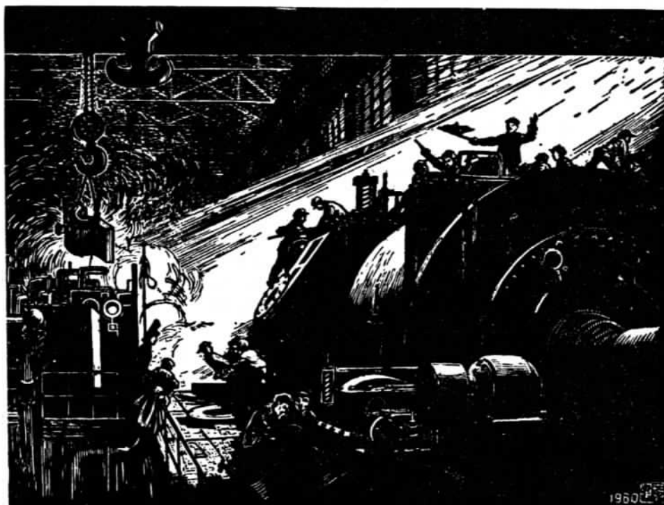
Installing a Generator
