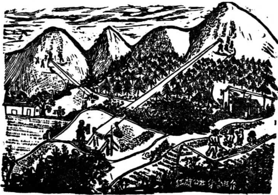
Overhead Cable Lines for Transport in a People's Commune
