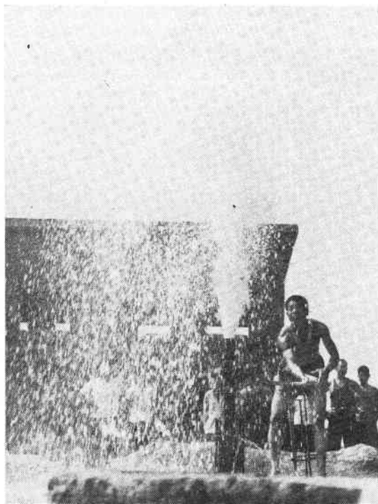
A thermal well sunk on the Huanghe delta by the Matou People's Commune. The water's temperature reaches 70 degrees centigrade.
