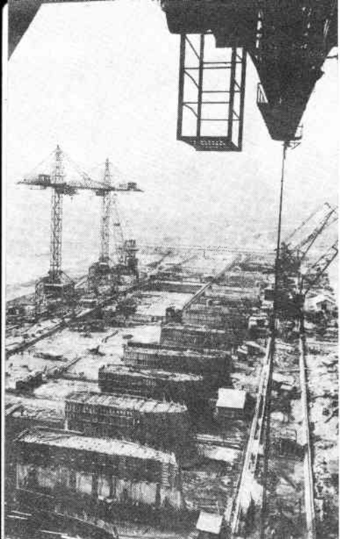
The 27-gate spillway in the center of Gezhou Dam.
