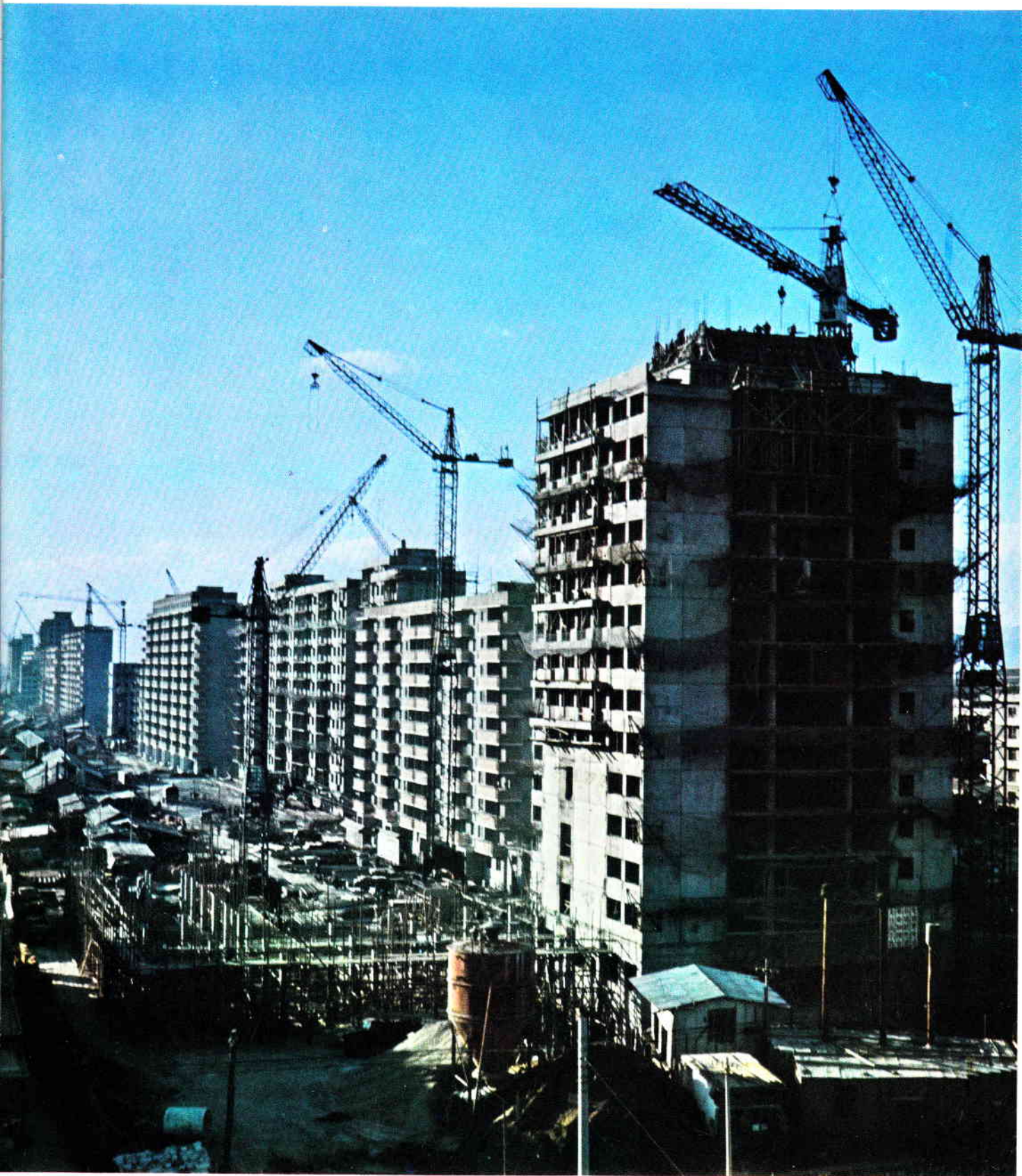
Residential building under construction.
