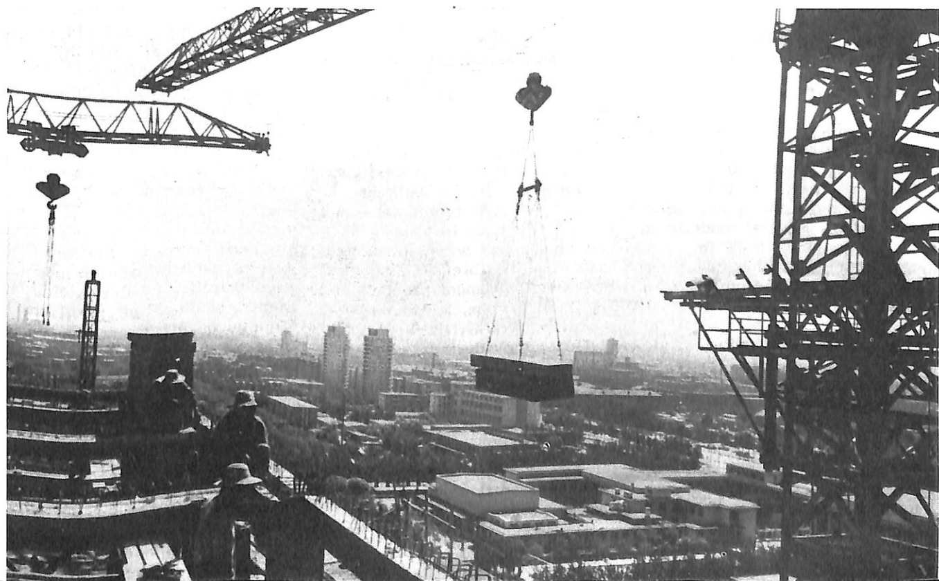
Building and construction work in Beijing.
