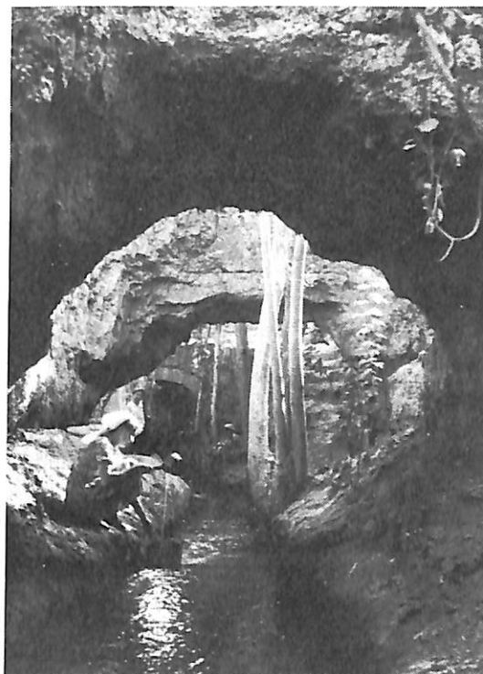
Karez, an underground channel for irrigation, traditional in Xinjiang. Cheng Zhishan
