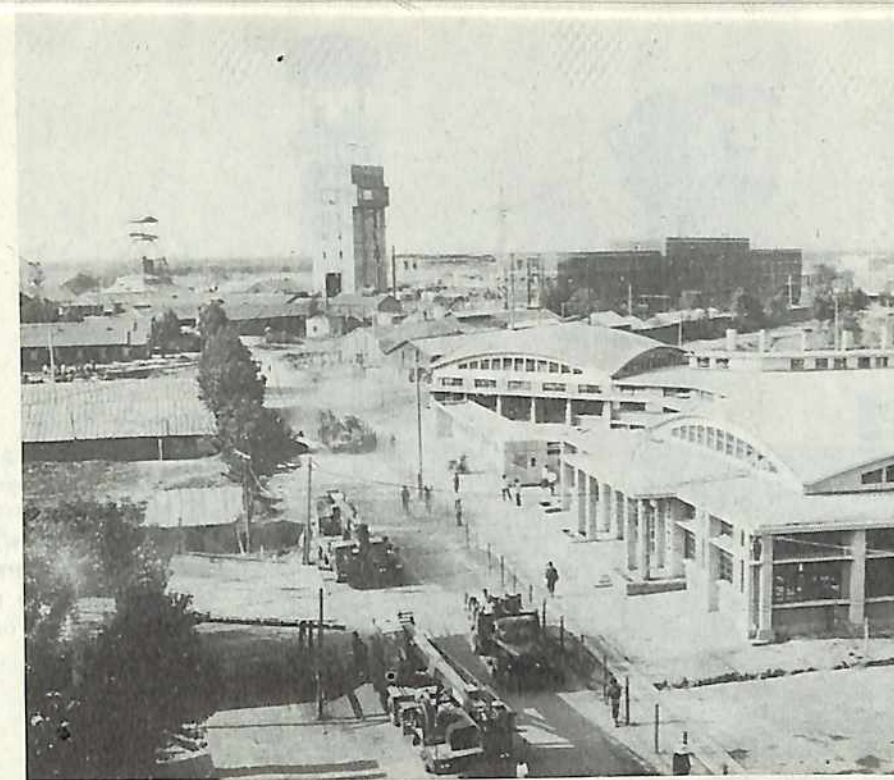
Xinglong mine under construction.
