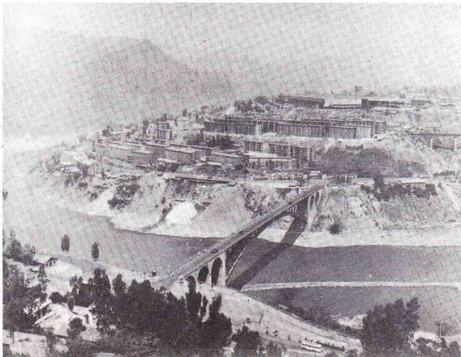
The iron and steel plant atop "the leveling."
