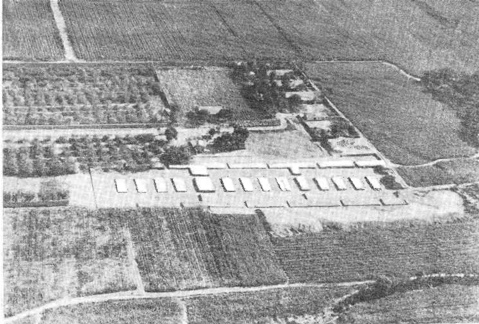
Excavation site, Building No. 7.
