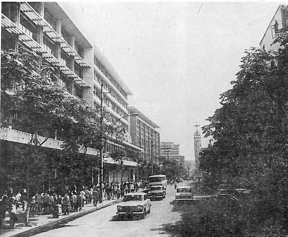
New buildings around the Monument to Liberation.
