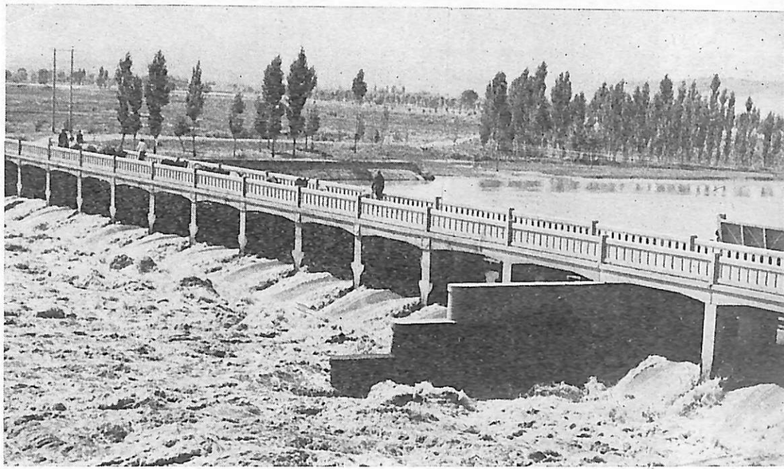
The Tanglai Canal which diverts water from the Yellow River for irrigation is one of the many projects to harness the river.
