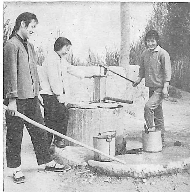
A covered storage well for drinking water.
