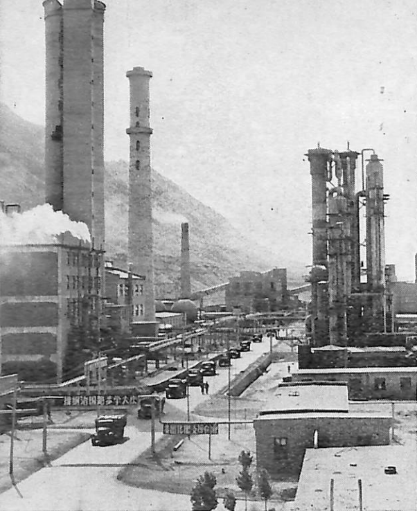
The newly-built Ula Chemical Fertilizer Plant.
