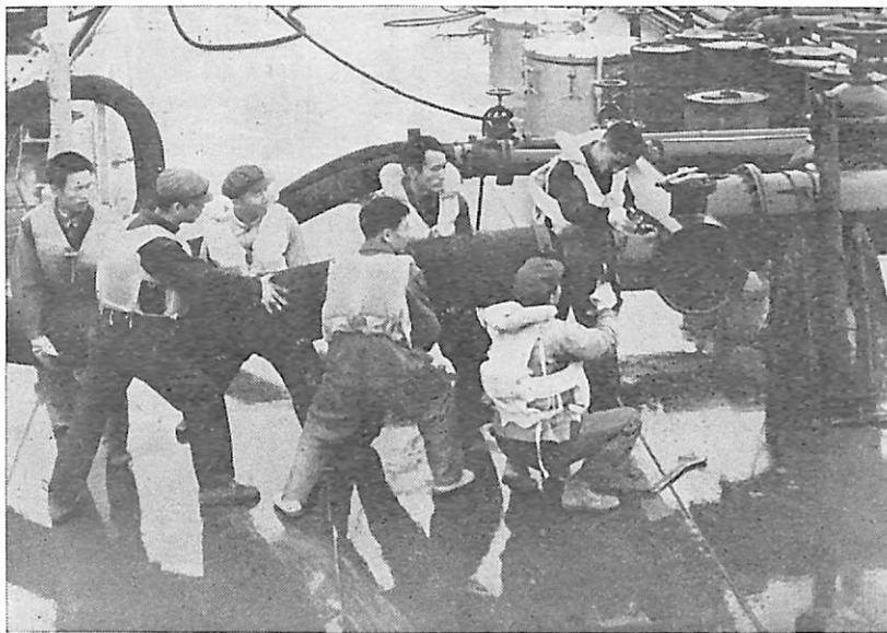
Getting the pipes ready for unloading crude oil.
