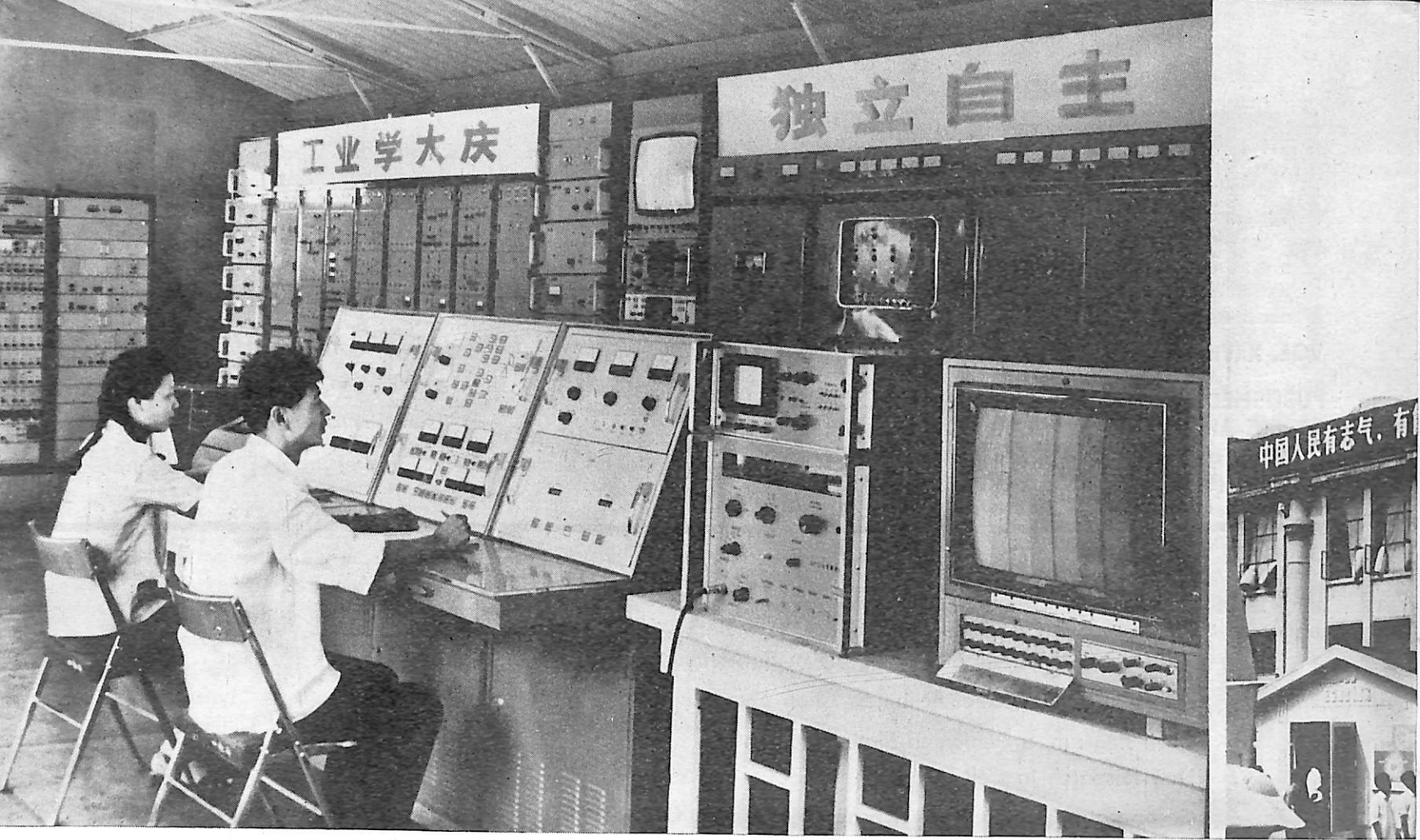
A satellite communications ground station, made in China.
