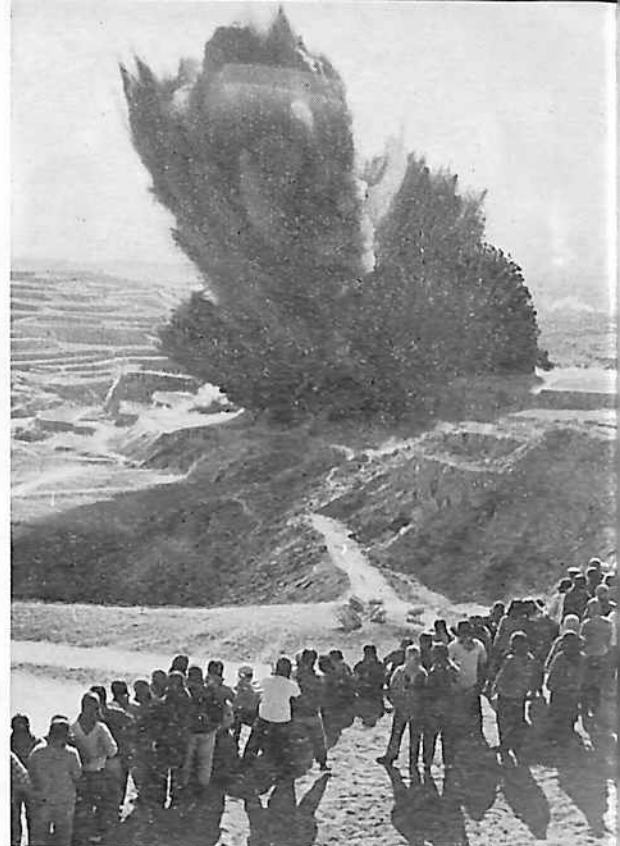
Changing mountains by directional blasting.
