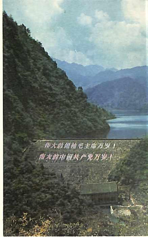
A hydropower station in the Chingkang Mountains.
