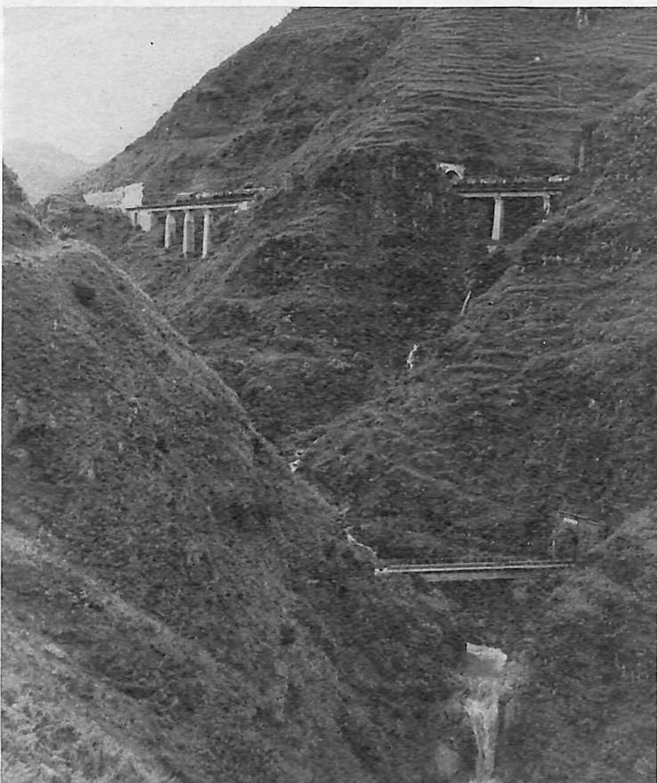
A continuous tunnel-and-bridge section of the Kweiyang-Kunming line.
