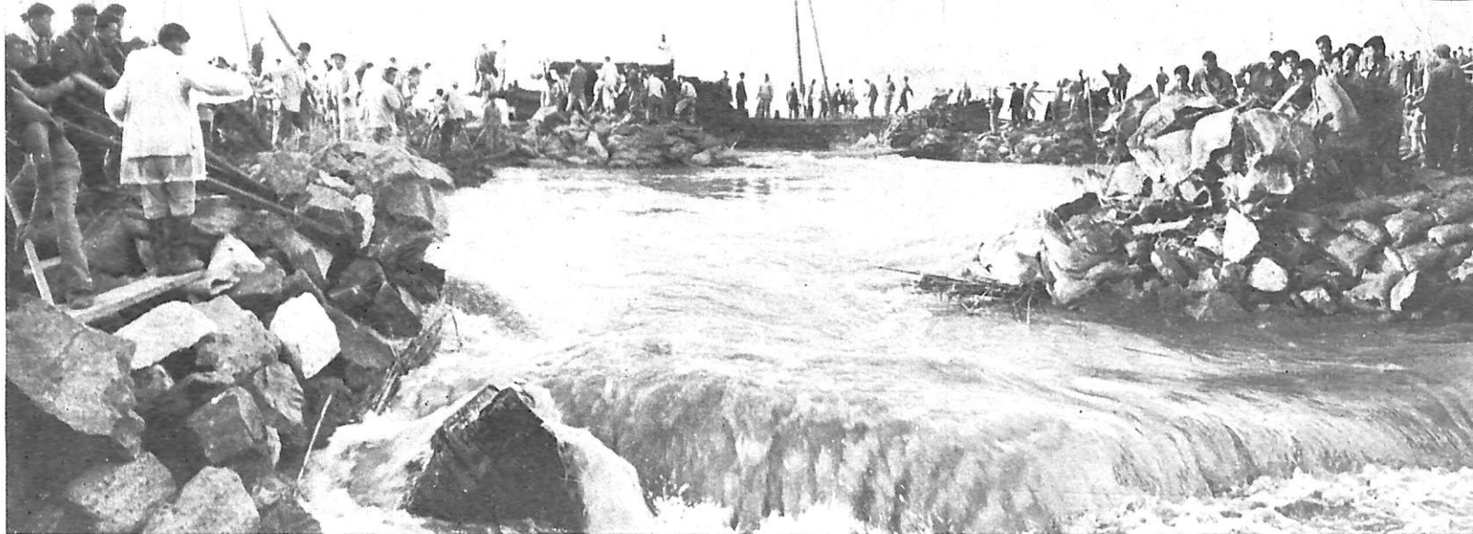
Over 30,000 peasants from 17 communes built the dyke for the Hsinchien Farm in the winter of 1971.
