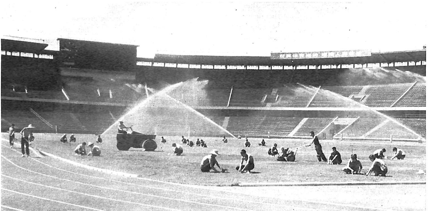
Preparing the Peking Workers' Stadium before a game.
