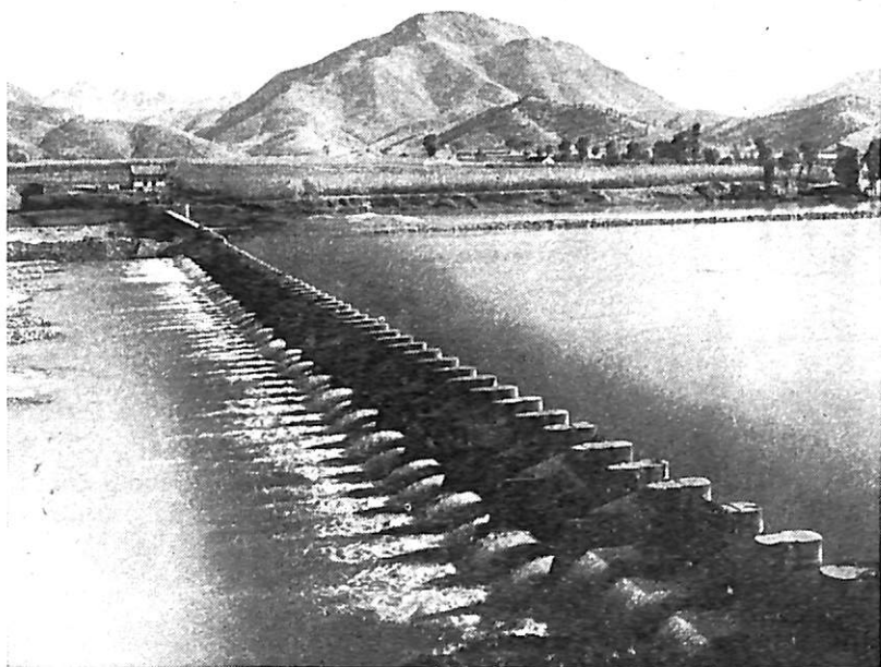
This dam of a commune power station gets its water by blocking an underground flow.
