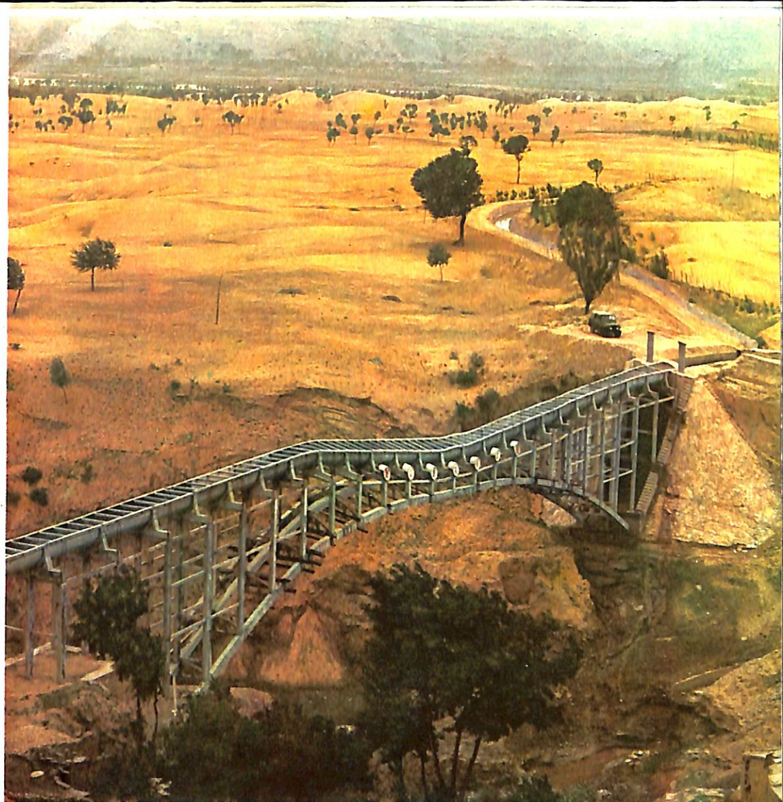
The newly-built 35-km. Yukao aqueduct brings water deep into the desert.
