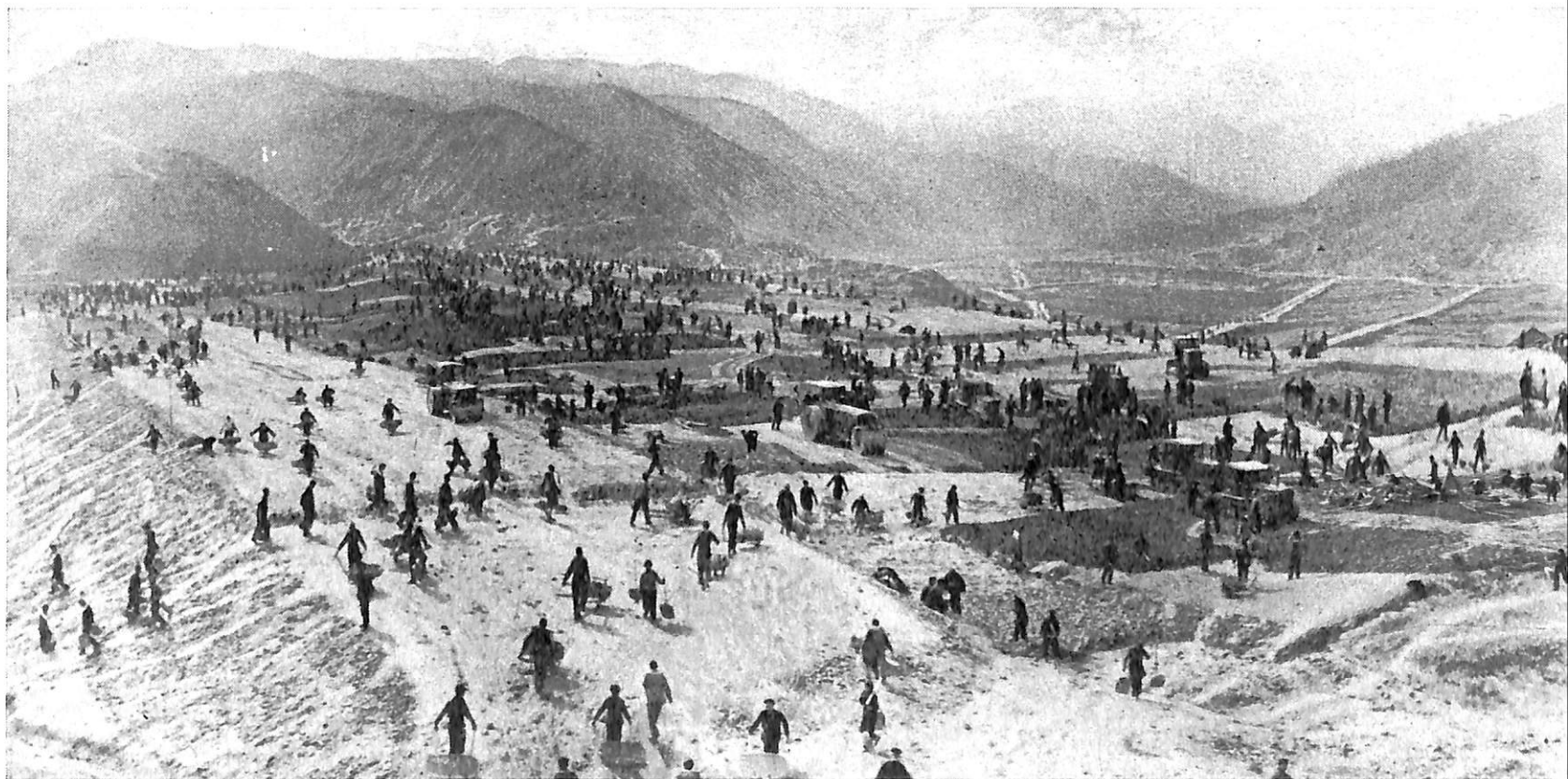
The worksite of a new reservoir.
