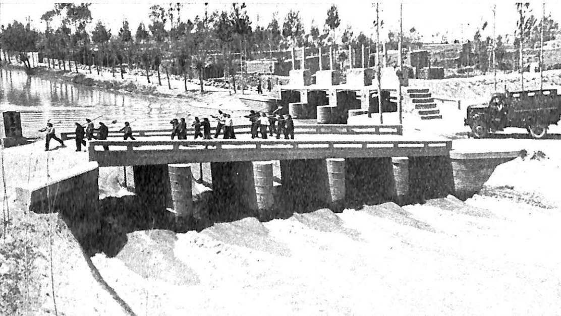
One of the many new bridges and sluice gates built in recent years.
