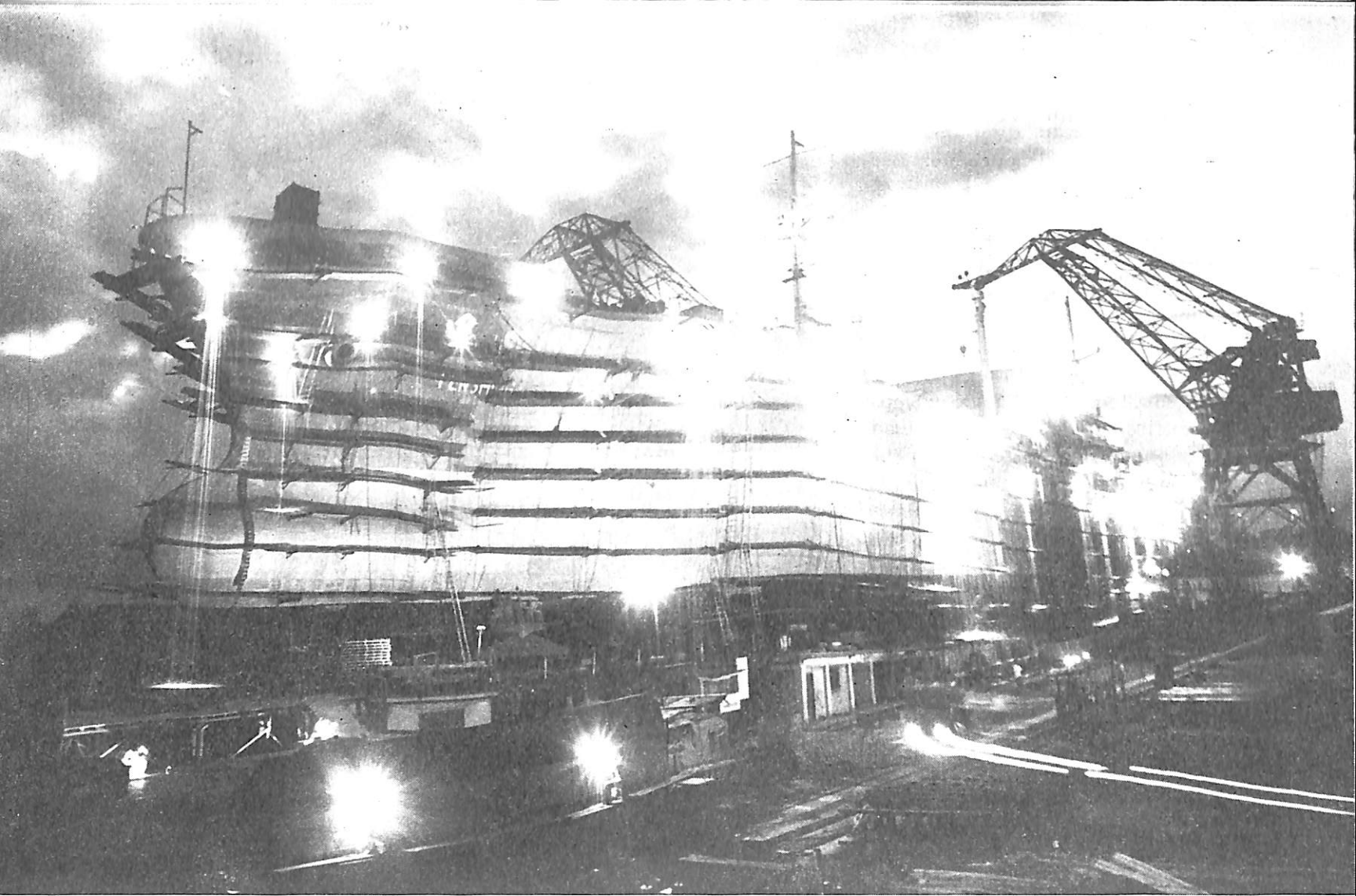
A 10,000-ton ship being built on 3,000-ton ways at the Shanghai Shipyard.
