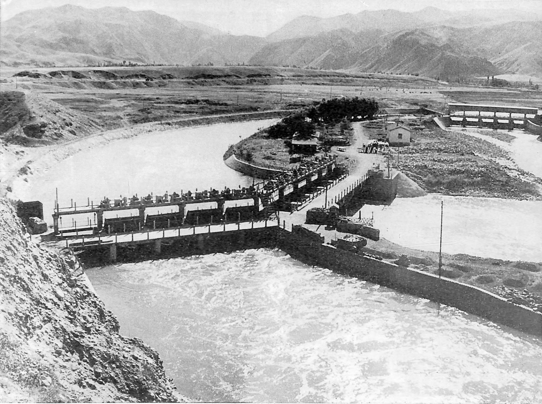
Water-control project for the Kashih irrigation district on the upper Ili River.
