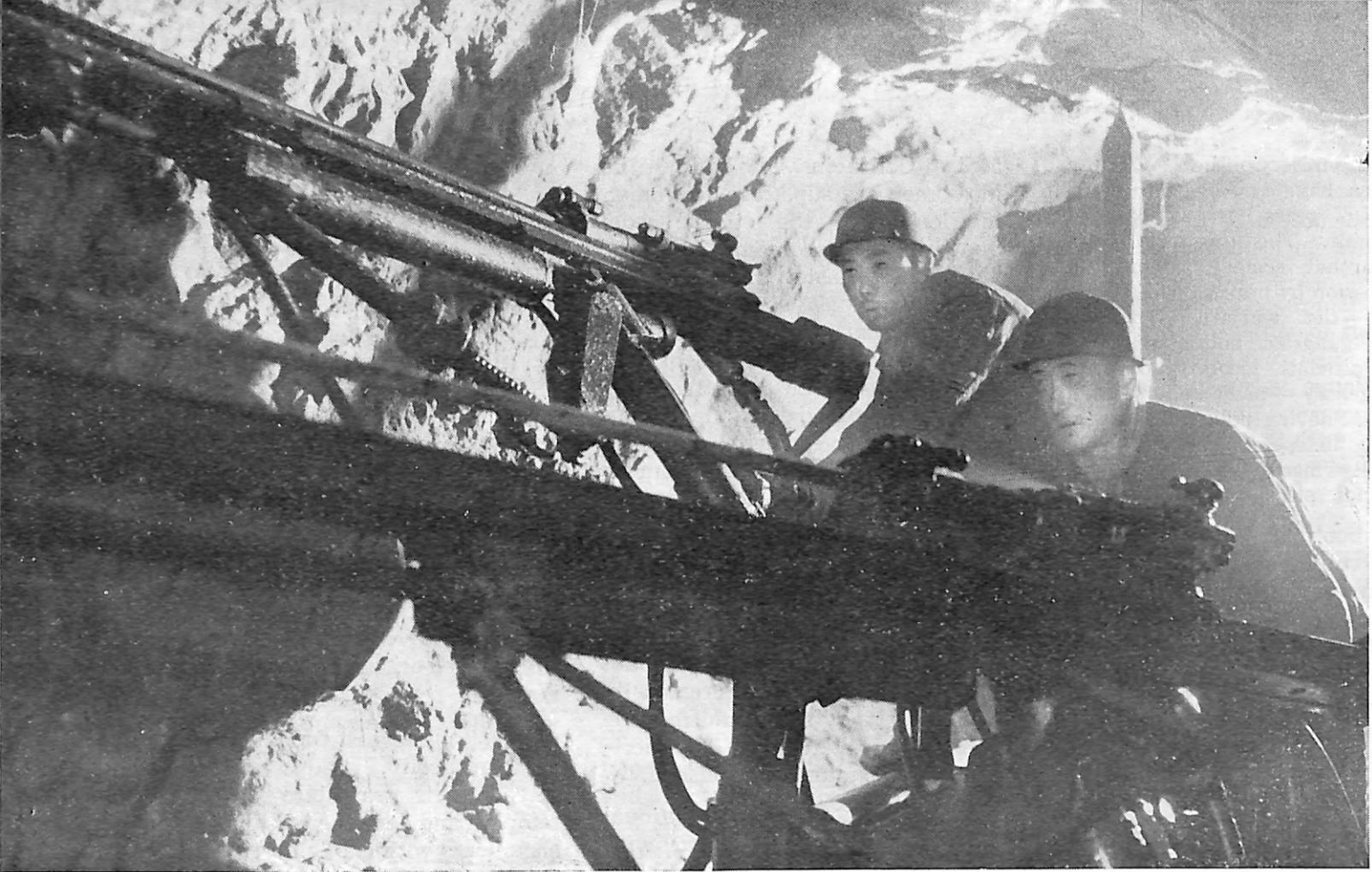
Twin-boom hydraulic drill car in operation.
