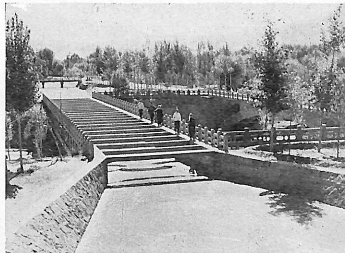
An aqueduct on a trunk canal that leads water from the Yellow River to the fields.
