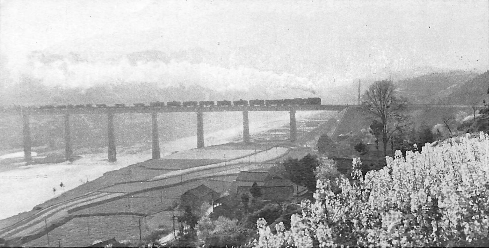
A freight train on the new line.
