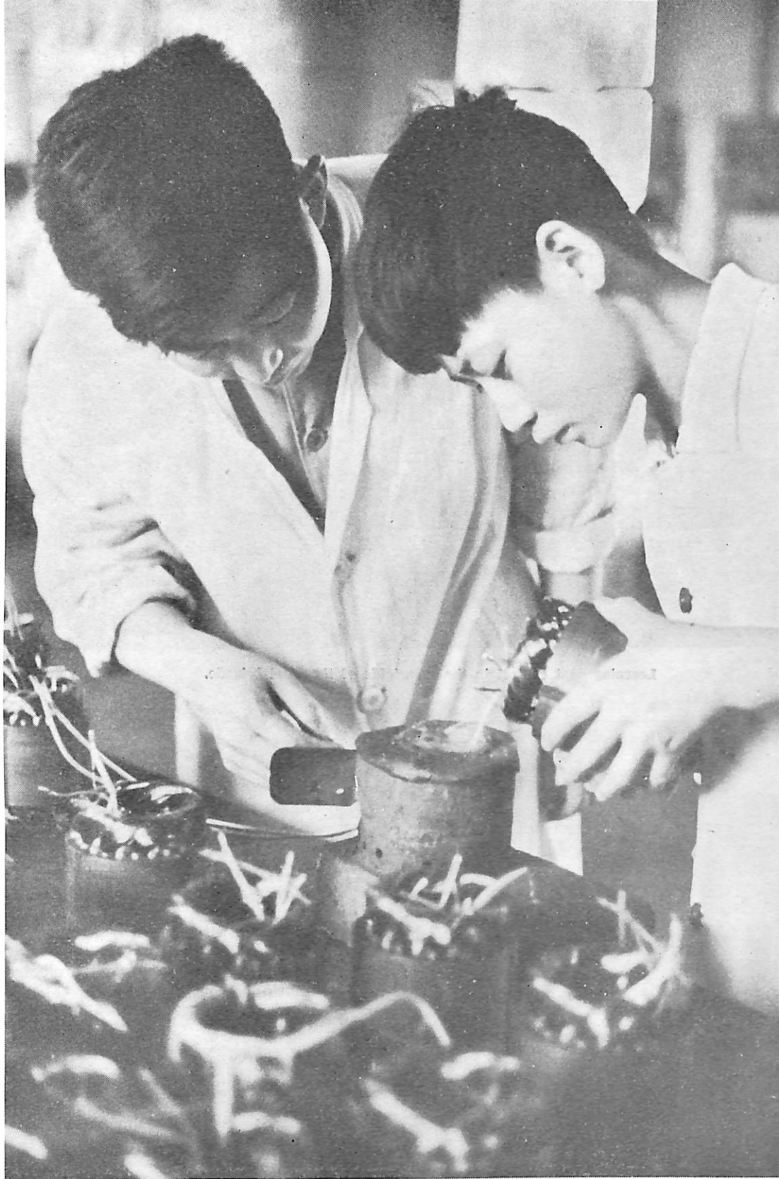
A student makes an assembly for a miniature motor with the help of a worker in the factory.
