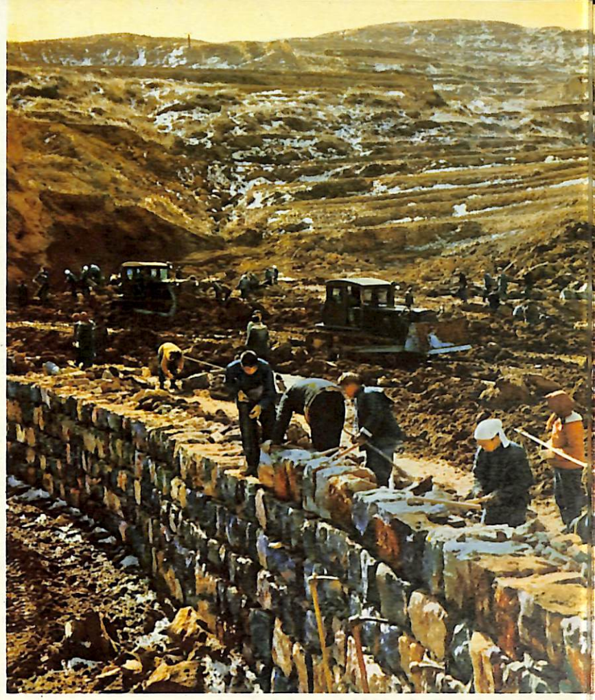
Building a stone wall for a terraced field.
