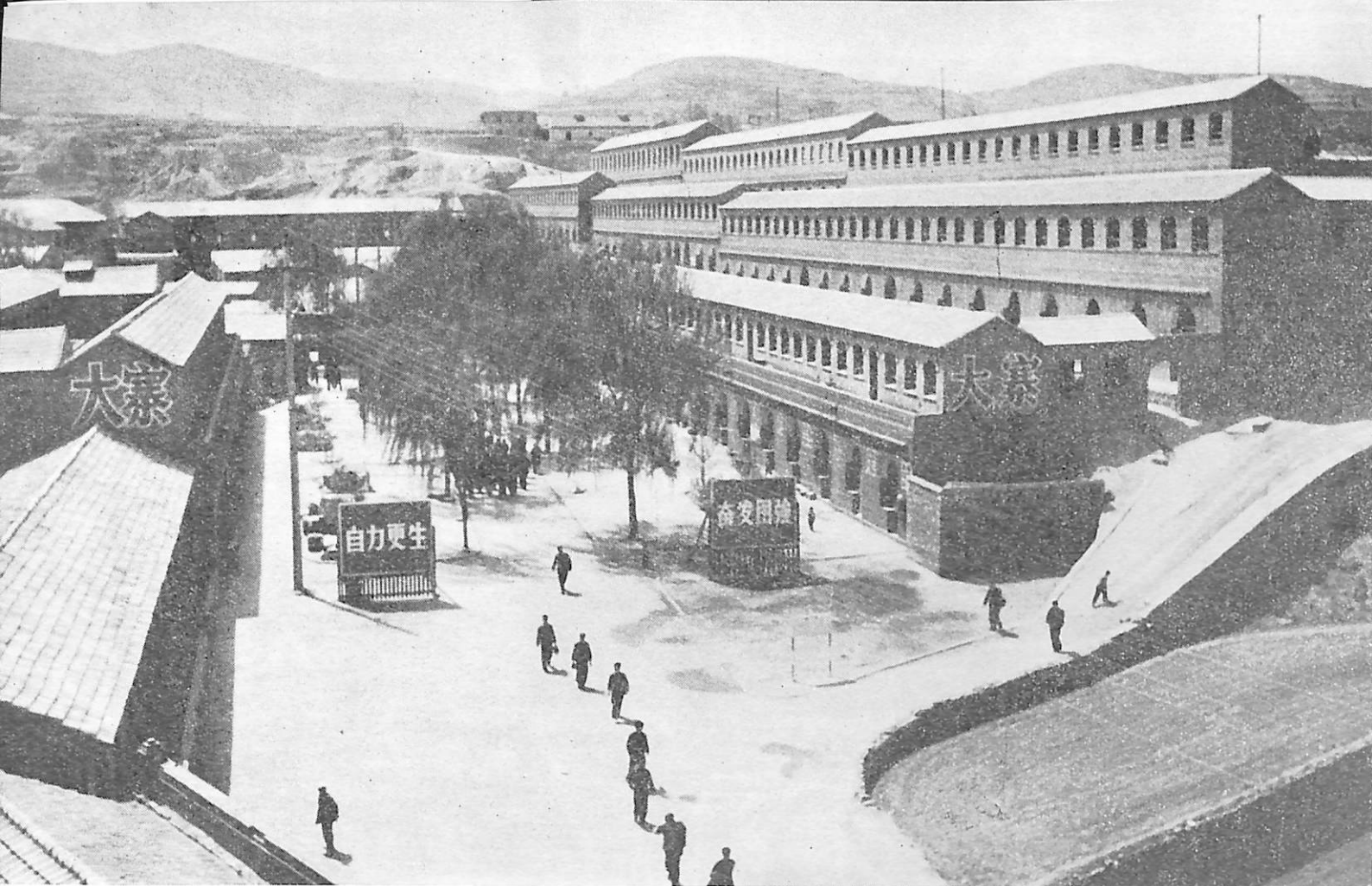
New homes for the Tachai peasants who used to live in rundown cave-dwellings.
