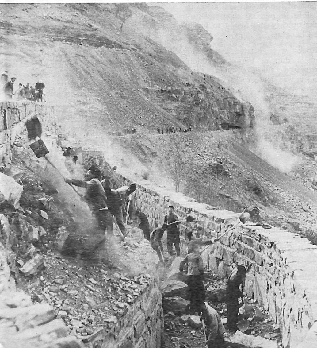
Work on the Tienchiao Canal.
