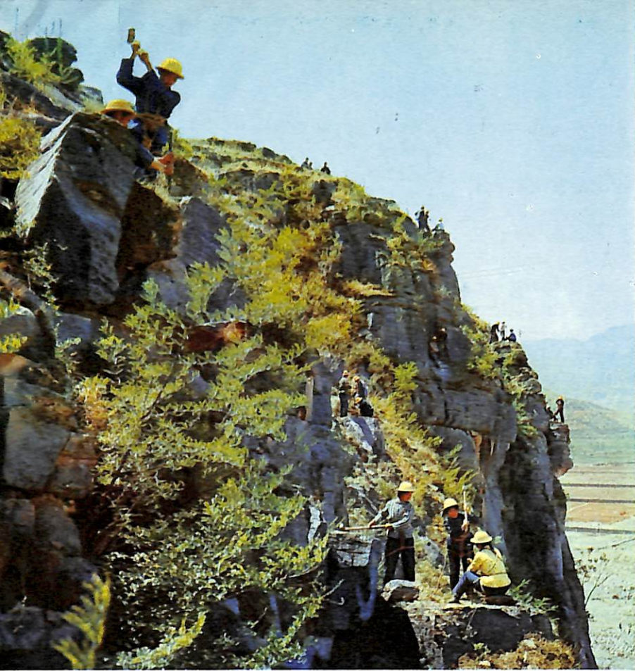
Stone for water conservation works is hewed out of the mountains.
