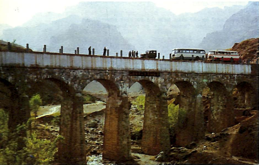
The 24-meter-high Taoyuanho aqueduct-bridge.
