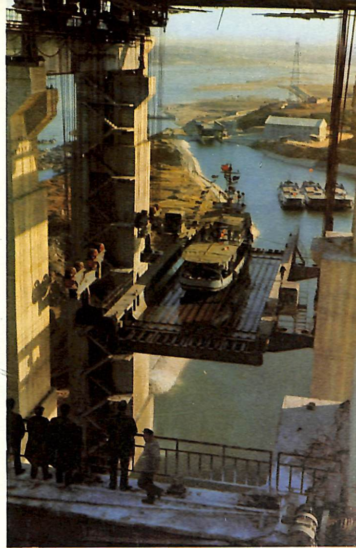
A China-made ship elevator takes a barge over the dam.
