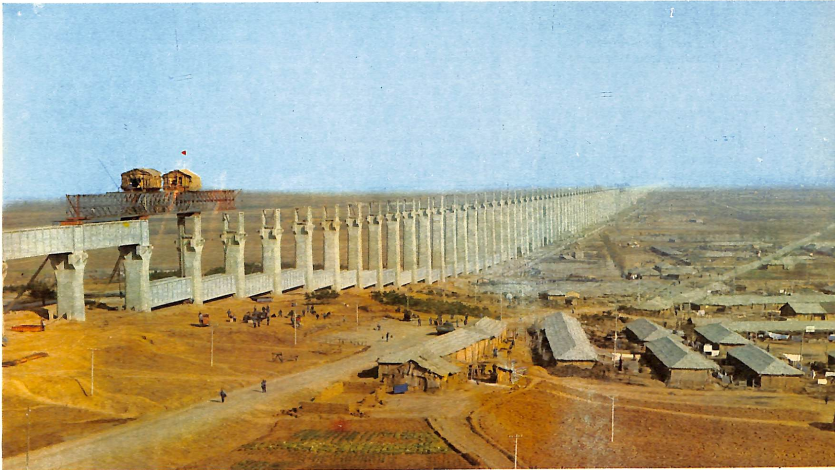
An aqueduct on the channel which will carry water from the Tanchiangkou reservoir to fields in Honan.
