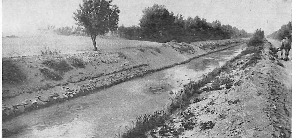
New irrigation system in Minchin county.
