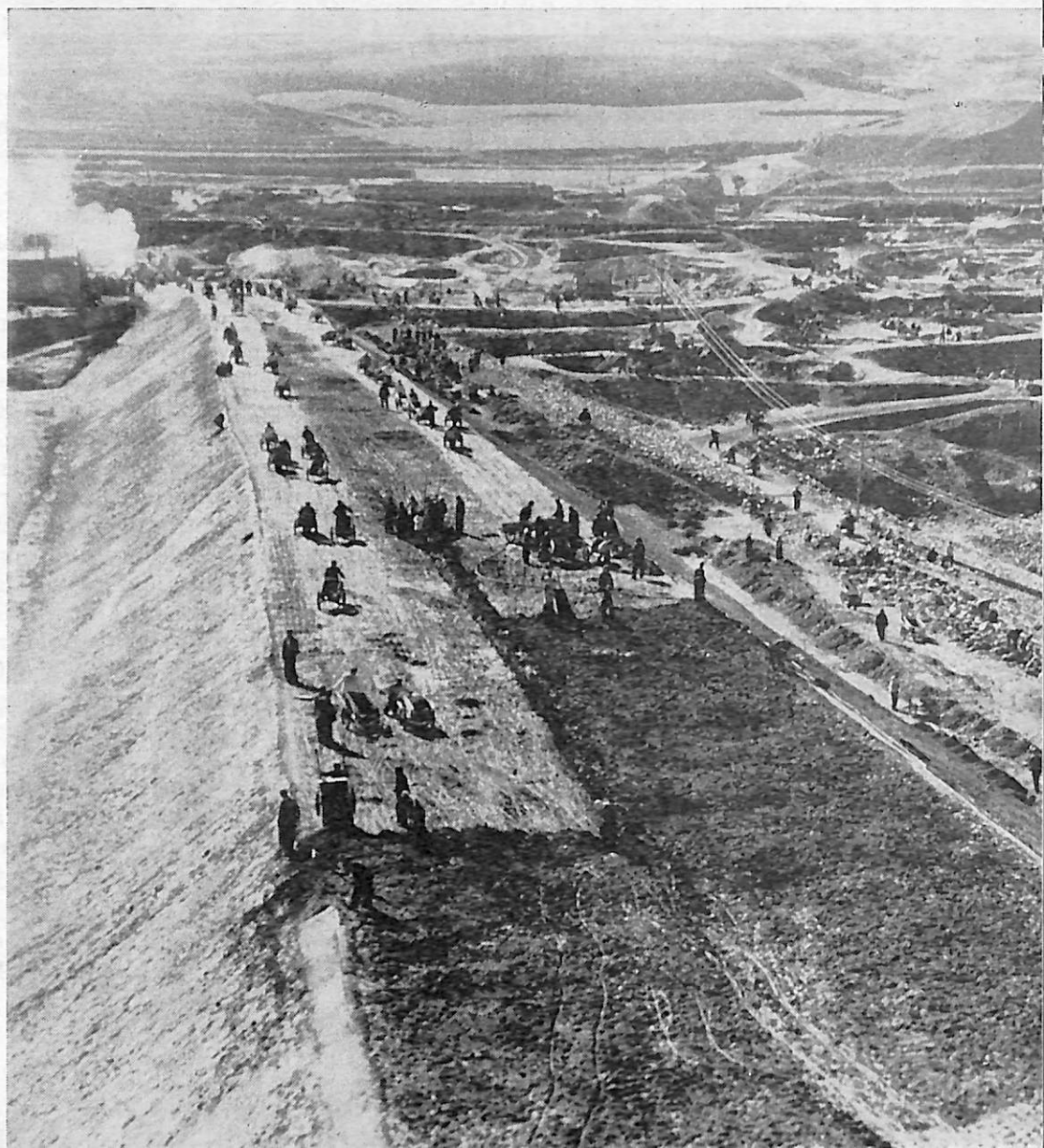
Tamaying dam in Shantan county under construction.
