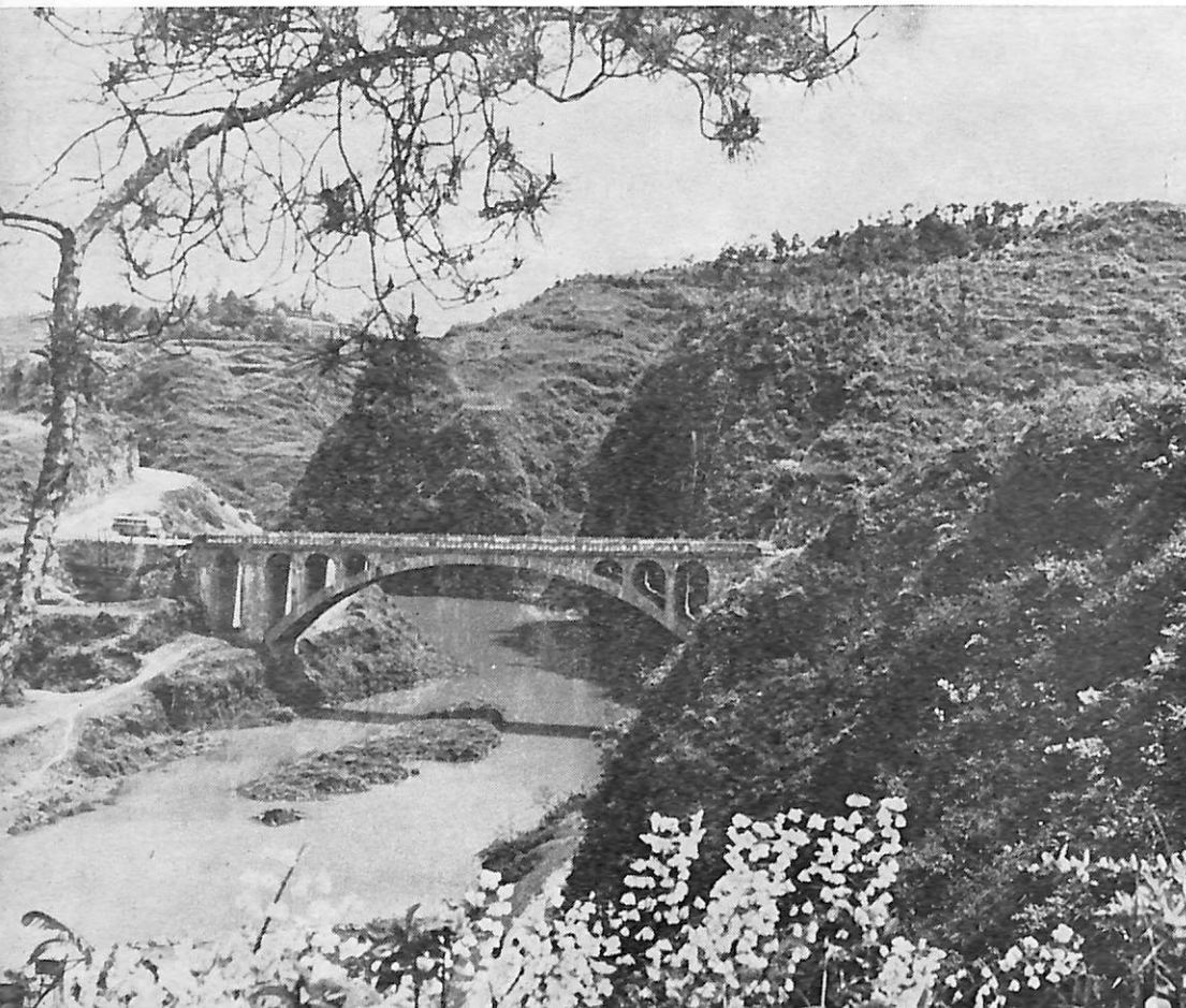
Road bridge in west Hunan.
