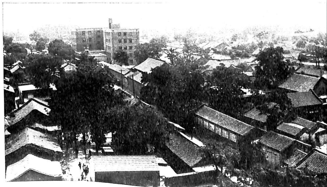
A section of the Fengsheng area in Peking.
