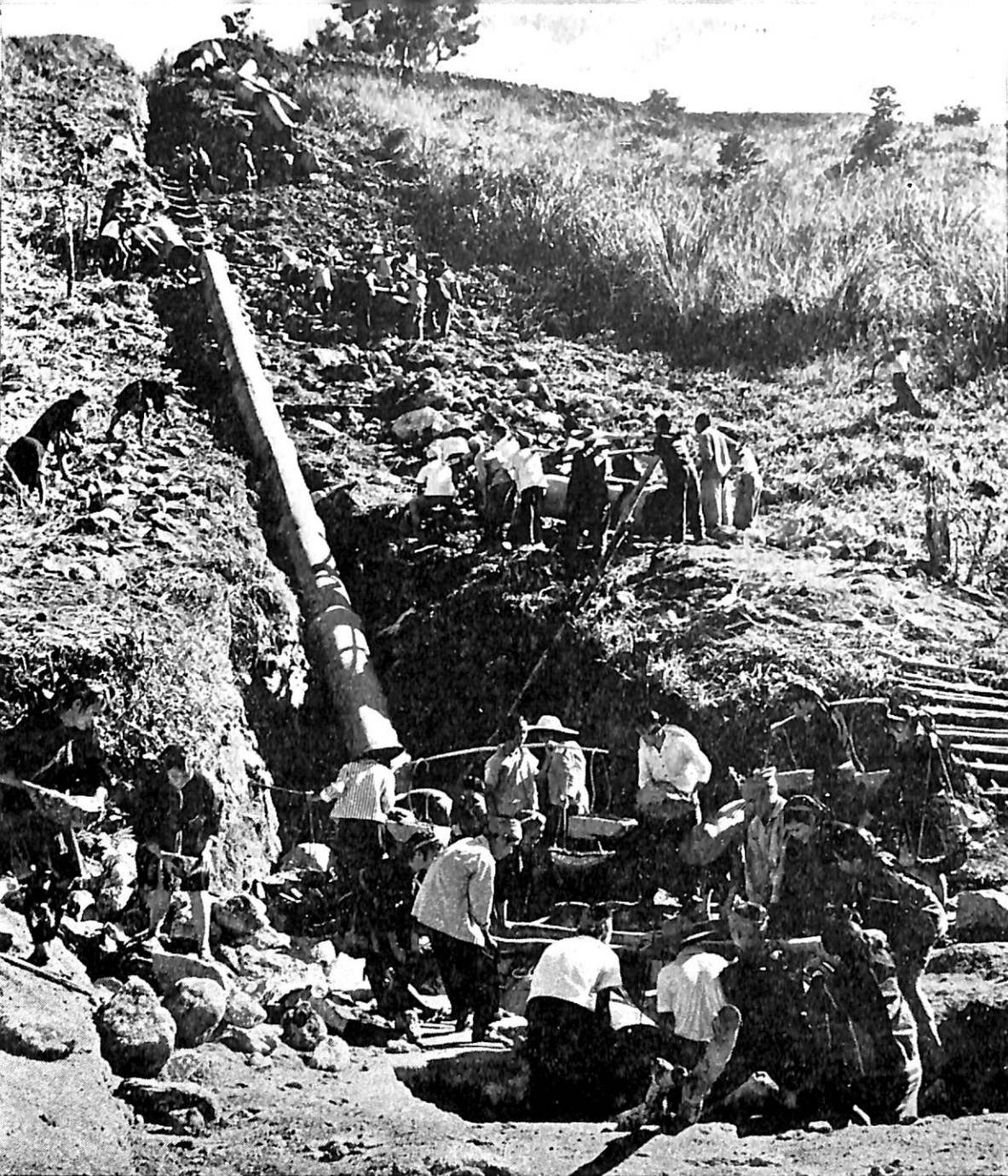
Hsin-an brigade members install pipe for a hydropower station.
