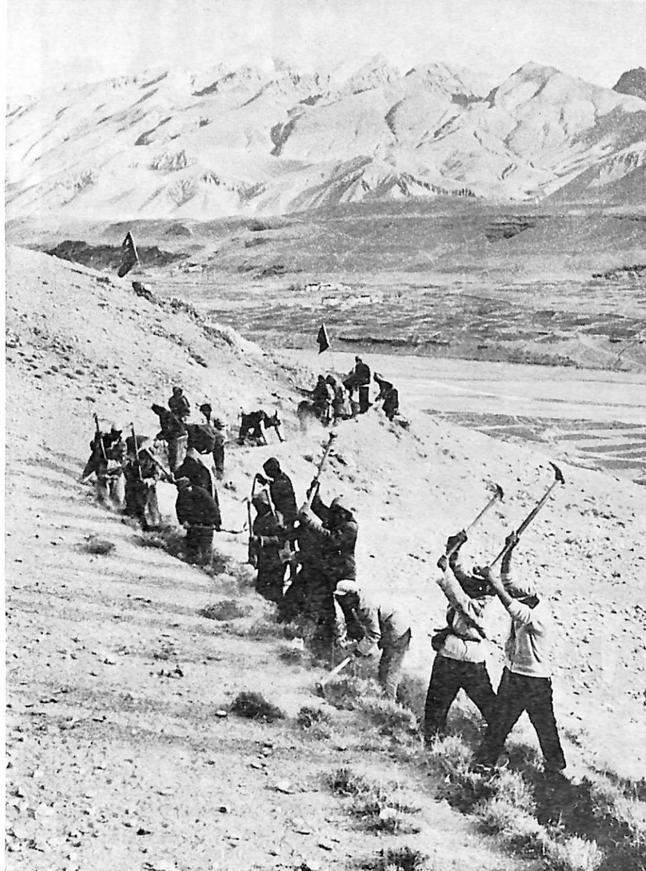
Digging ditches on the slopes.
