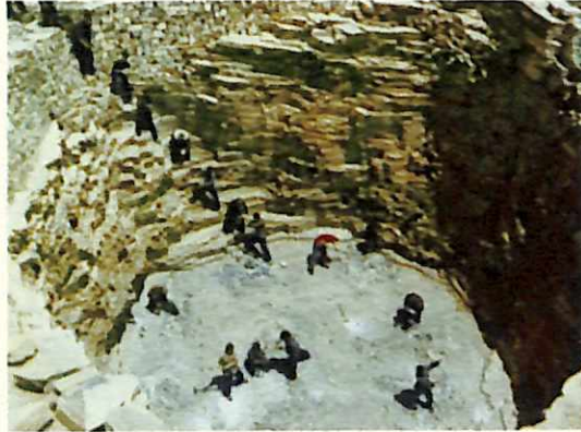
The cistern in progress.
