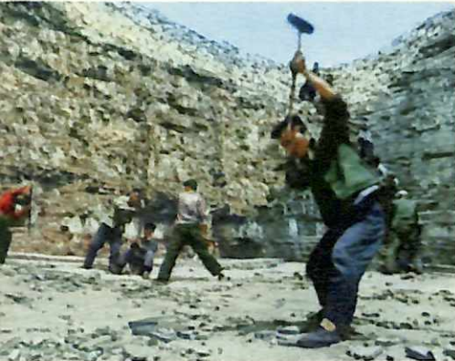
Work begins on hacking a cistern in the rock.
