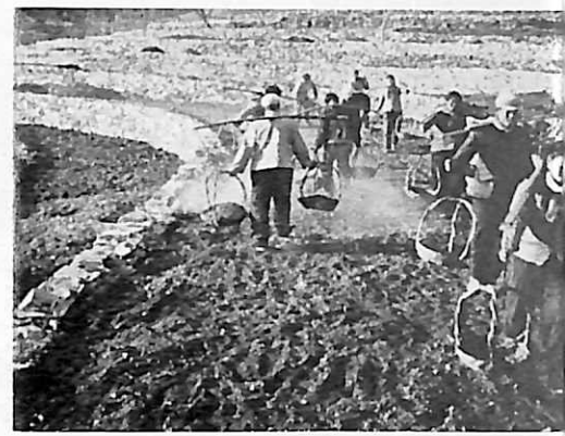
Adding another layer of earth.
