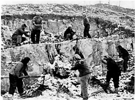
Digging out the terraces.
