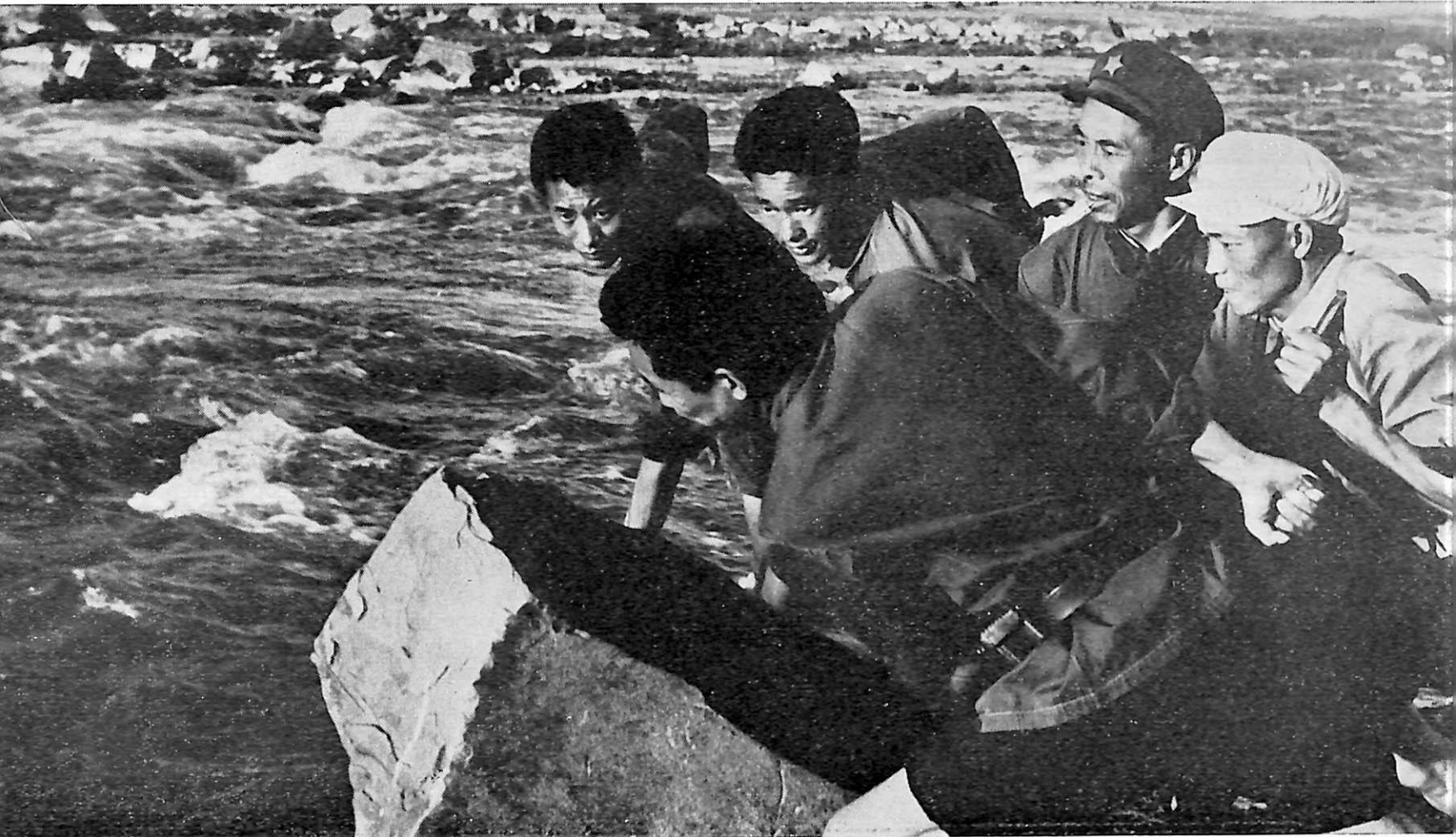
An armyman joins commune members in building a dam.
