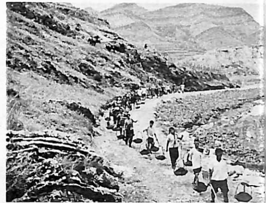
Transporting earth from the other side of the mountain.
