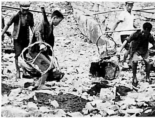
The earth is spread over the rock floor.
