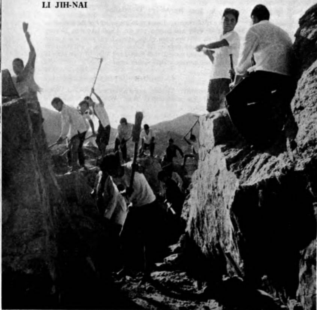
Splitting a mountain for a main irrigation canal across its face.
