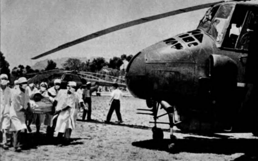
Army helicopters arrive to move injured workers to hospital.
