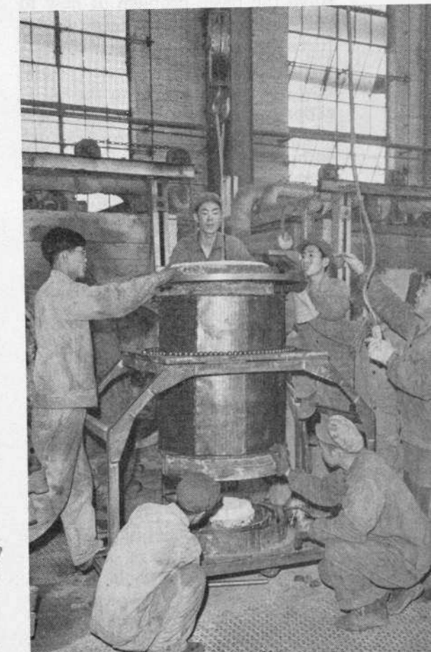
Members of the shock team installing a high-efficiency heating furnace.
