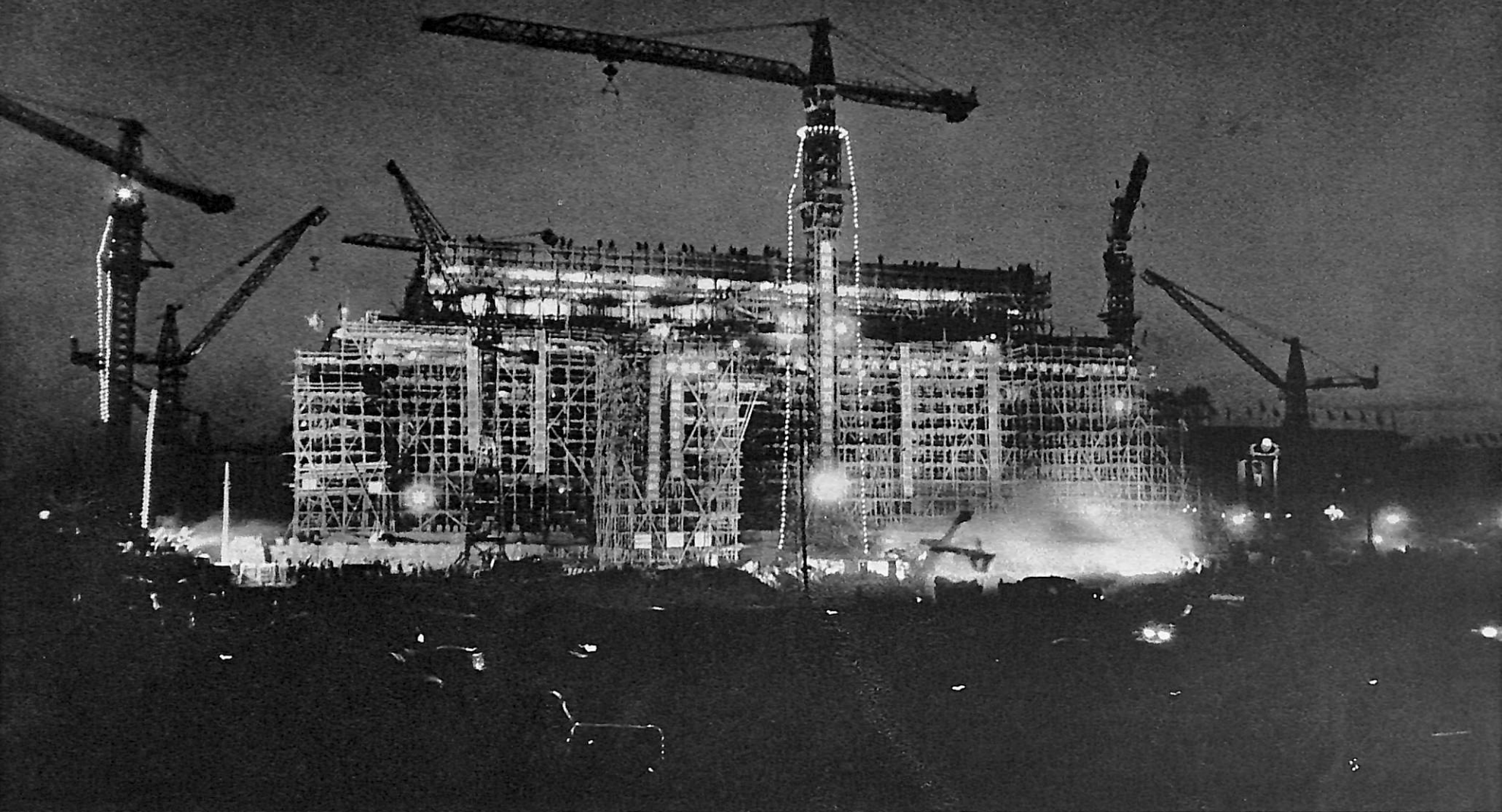
To complete the memorial hall as quickly as possible, work on the project goes on day and night.
