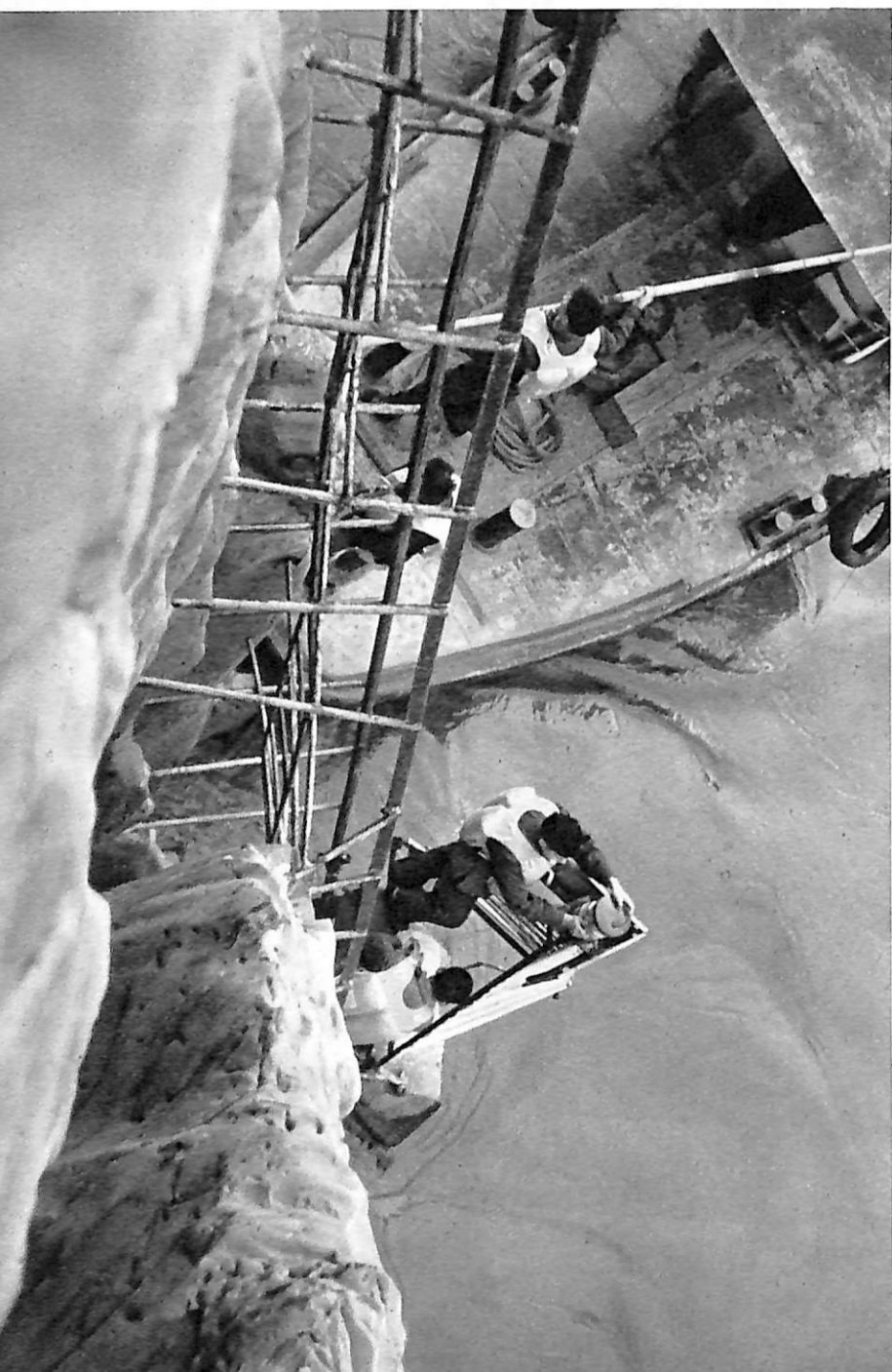
Checking and repairing a self-raising and lowering electric light.
