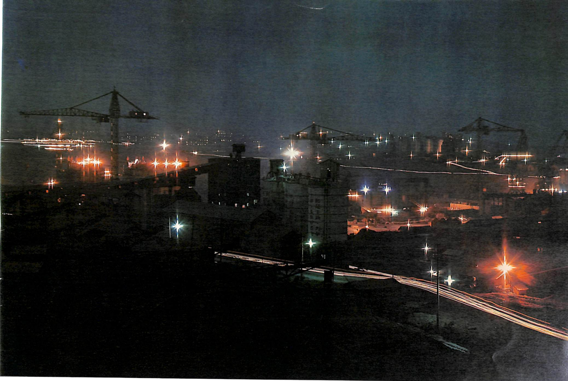
A construction site.
