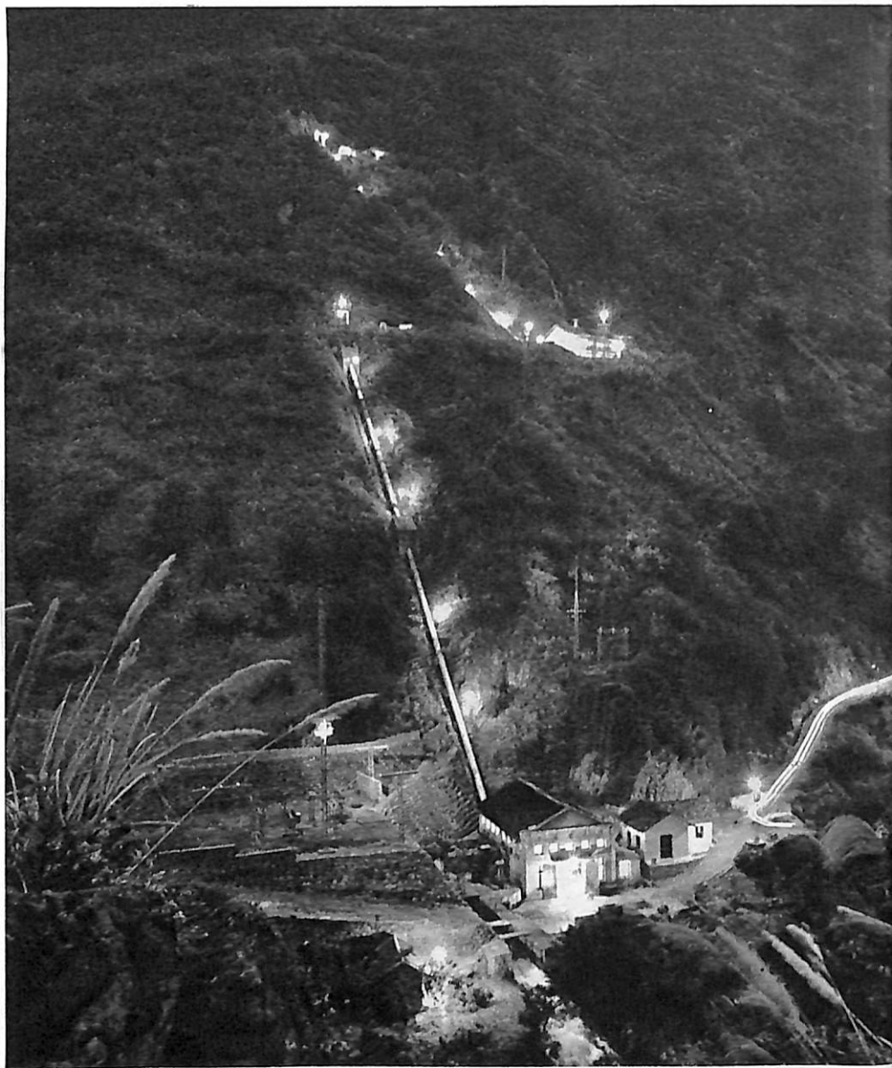
Rural construction goes ahead. A small hydropower station built by the people of Patung County on the Wanfu River.
