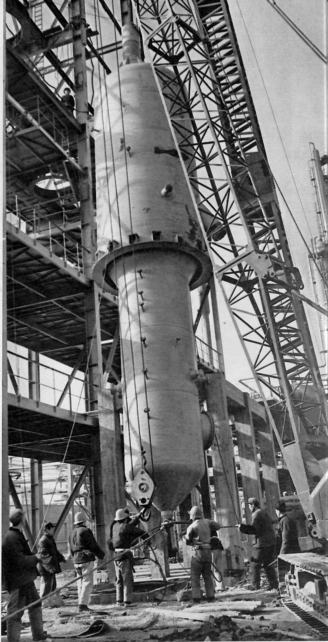
The second stage of the project under construction.
