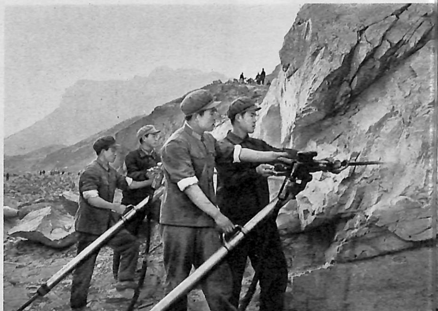
Digging a tunnel.
