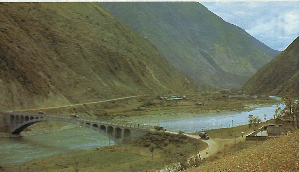
The new Luting Bridge.
