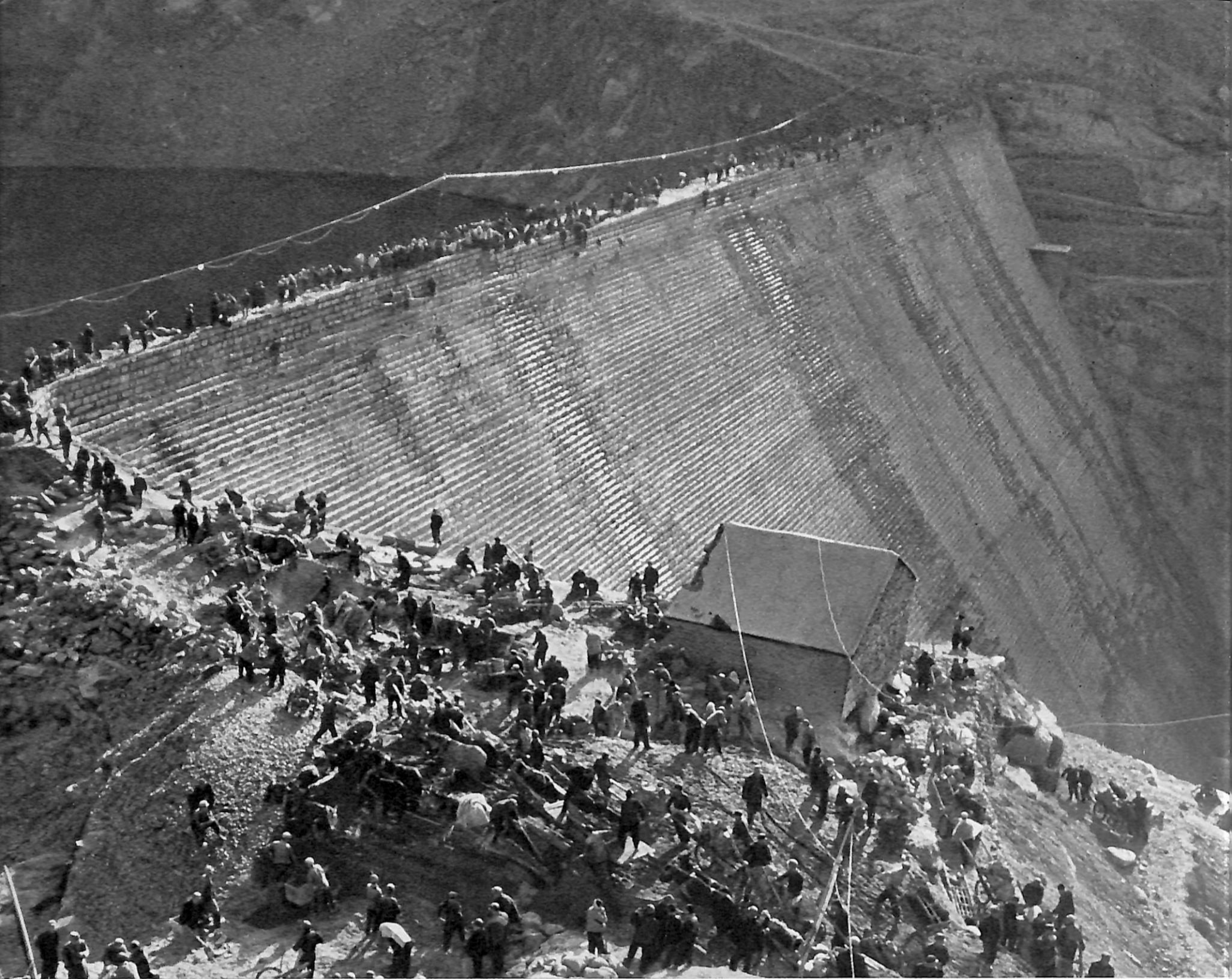
Constructing a reservoir.
