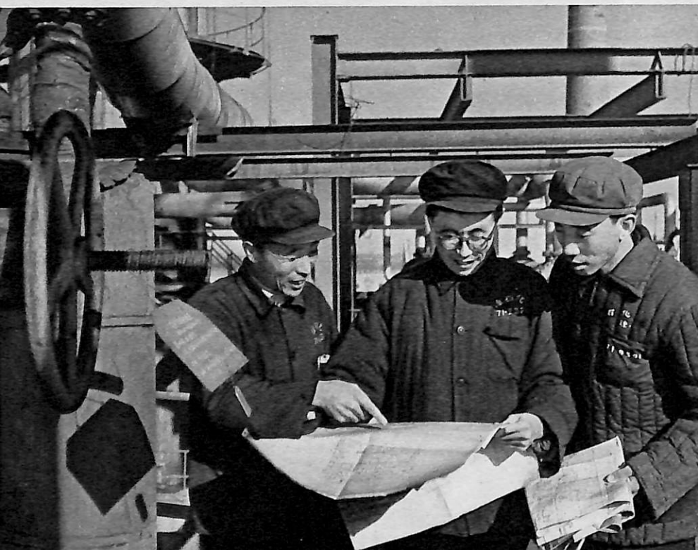
Thanks to technical innovations by workers in the processing and machine-repair workshops, production of the vacuum distillation unit now is more than twice designed capacity. Here a worker (right), a technician (centre) and a cadre are discussing how to tap latent production potential.
