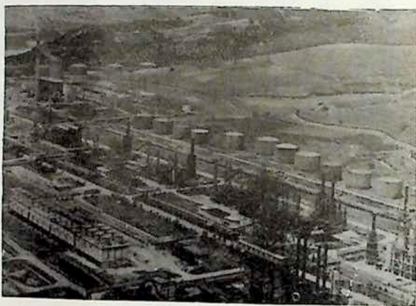
The oil-processing plant at Ballsh
