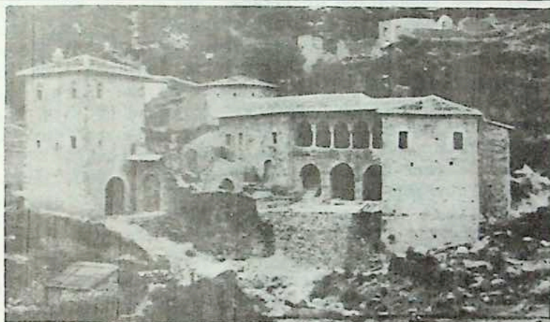
The Fortress of Dukat after Restoration
