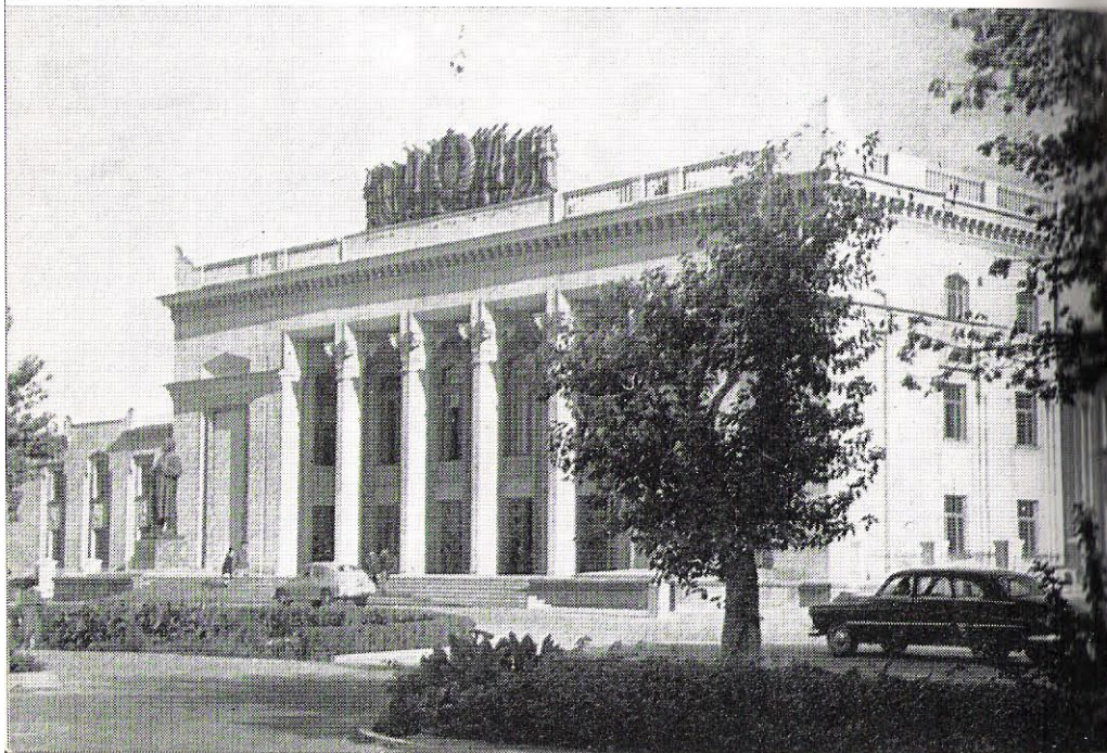
The Supreme Soviet and the Council of Ministers of the Turkmen Republic are housed in the building below.
