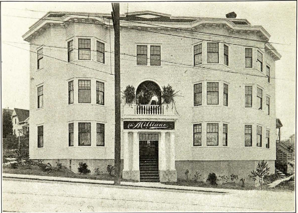
MR. CHANDLER'S 12-FAMILY APARTMENT HOUSE, SEATTLE.
