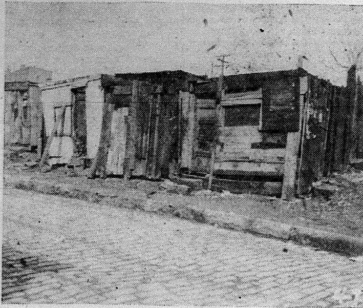
Photo shows type of houses Negro families are forced to live in after slaving long hours in the field and factory.
