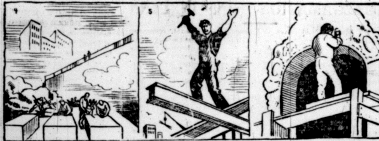
4—The unimportant men who lay the foundation after the stone has been quarried and transported by others just as unimportant and common. 5—The mere wage earner who risks his life in mid-air with the steel girders, made by unimportant steel workers. 6—The man who carves the stone that gives beauty to the structure—just a humble laborer.—(D—)
