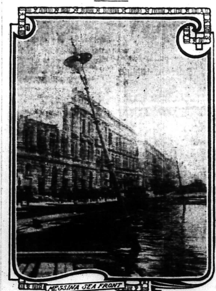
This photograph of the sea front at Messina shows how the sturdy stone building that faced the strand in a ground along the sea front caused the sea to cover the wide strand that formerly lay between the line of buildings and the shipping wharfs.
